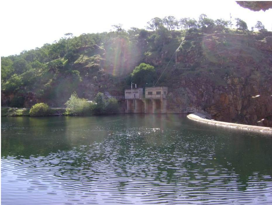
**Figure 3.4.3-2** TID diversion tunnel entrance on left bank.
