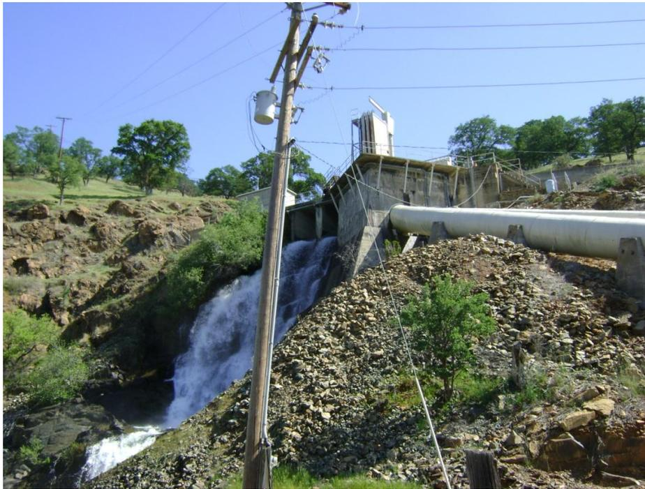
**Figure 3.4.4-1 TID forebay and penstock intake. Flow is being discharged at the forebay sluice gates.**
