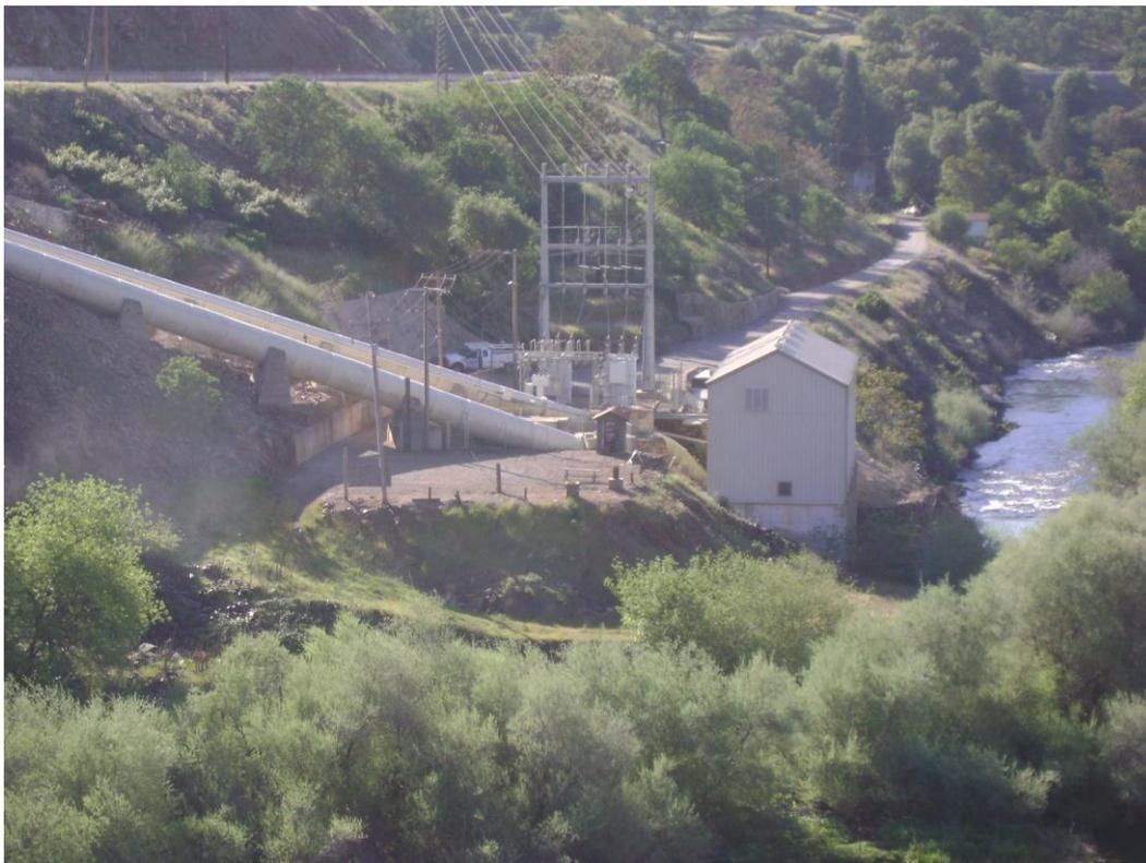
**Figure 3.4.6-1 Penstock, powerhouse, tailrace, and switchyard.**
