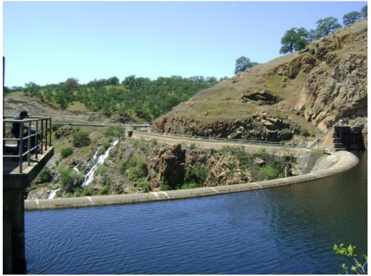
Figure 3.4.1-2La Grange diversion dam from TID intake on left bank.<br/>Note water flow from MID old canal to river below.
