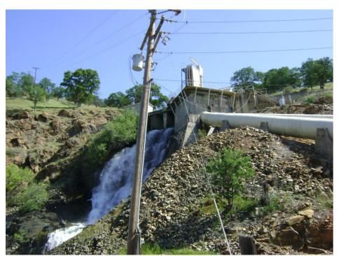
Figure 3.4.4-1 TID forebay and penstock intake. Flow is being discharged at the forebay sluice gates.
