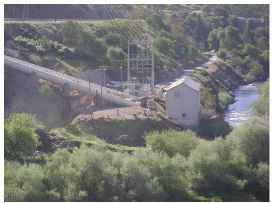
Figure 3.4.6-1 Penstock, powerhouse, tailrace, and switchyard.
