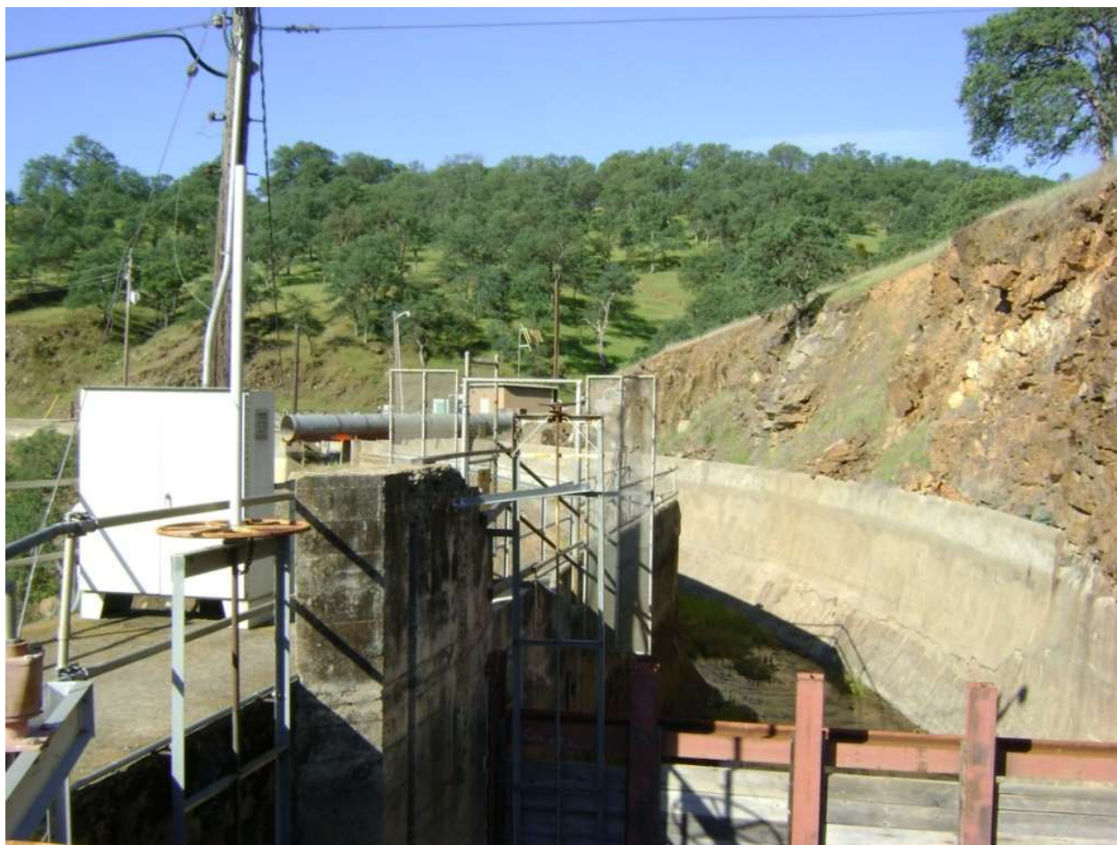
Figure 2.3-1. Retired MID main canal on west (right) bank. Gate stems and hand-wheels controlling the openings of the gates that pass flow to the hill-side release are seen in the far left of the photo.
