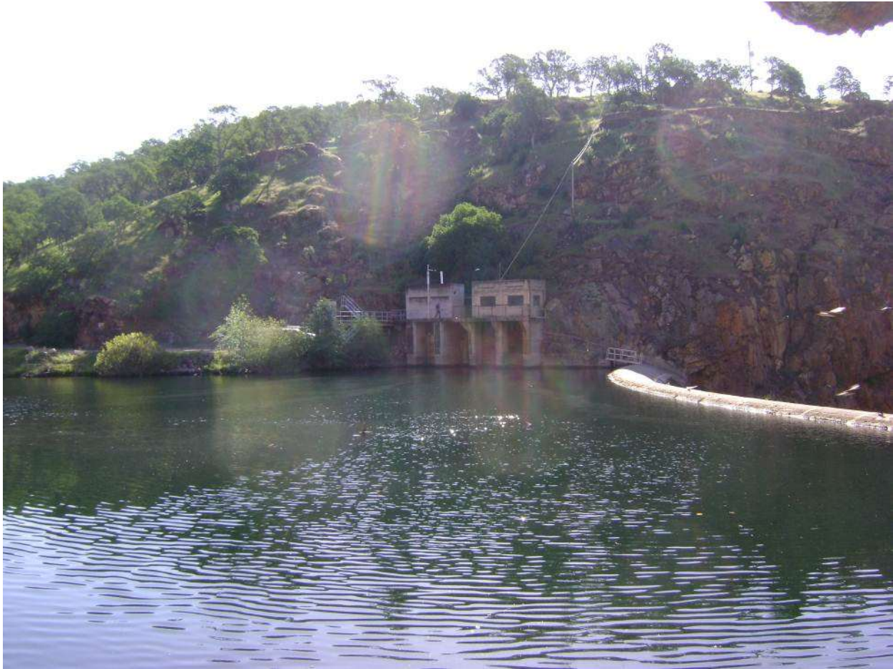
Figure 2.3-2. TID diversion tunnel intake on east (left) bank.
