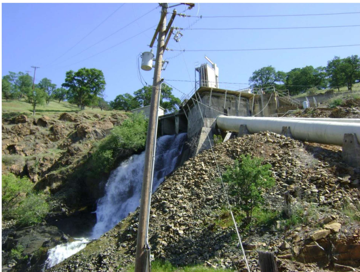
Figure 2.4-1. TID forebay and penstock intake. In the photo, flow is being discharged at the forebay sluice gates.
