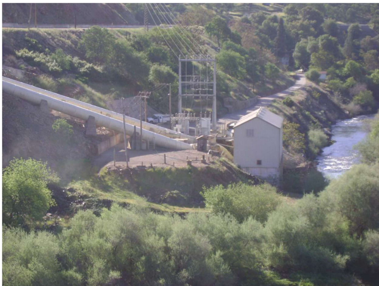
Figure 2.5-1. View looking downstream of TID’s penstocks, powerhouse, tailrace, and substation.
