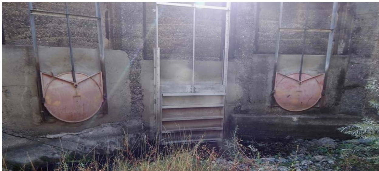
**Figure 3.0-1. Hillside valves which pass flow from the MID canal to the plunge pool below LGDD.**
