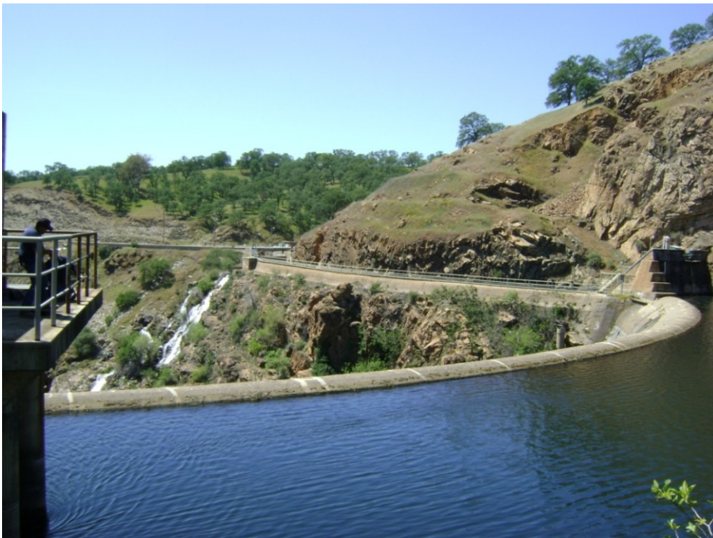
Figure 2.1-3. La Grange Diversion Dam from TID intake on left bank. Note water flowing from MID Hillside outlet to river below.
