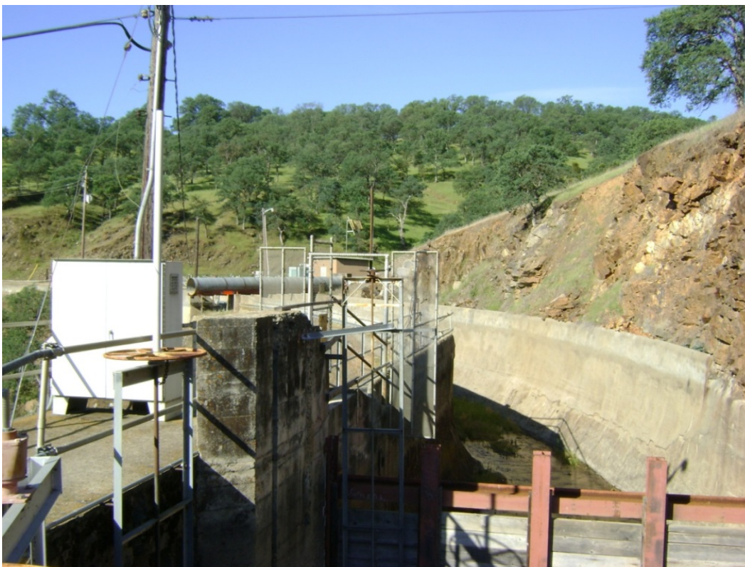
Figure 2.3-1. Retired MID main canal on west (right) bank. Gate stems and hand-wheels controlling the openings of the Hillside gates that pass flow to the plunge pool below LGDD are seen in the far left of the photo.
