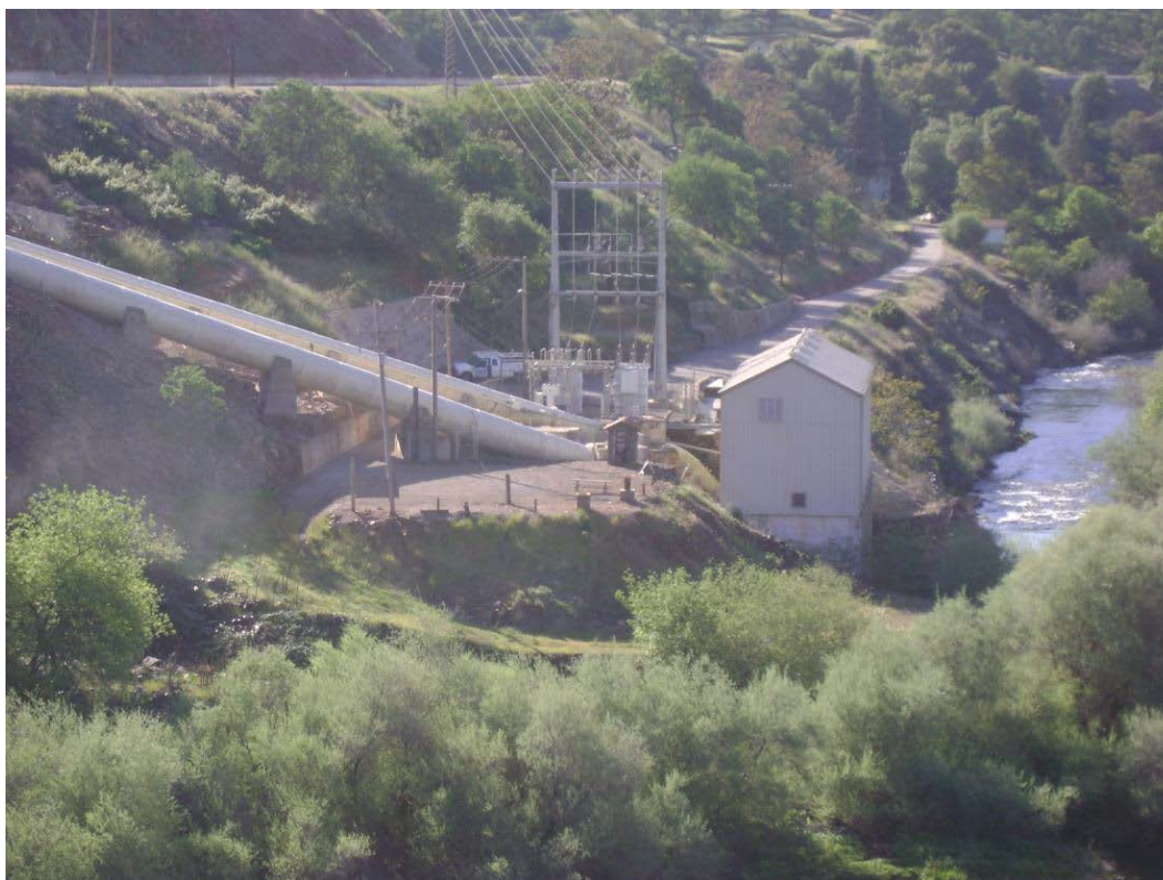
Figure 2.5-1. View of TID's penstocks, powerhouse, tailrace, and substation looking downstream.
