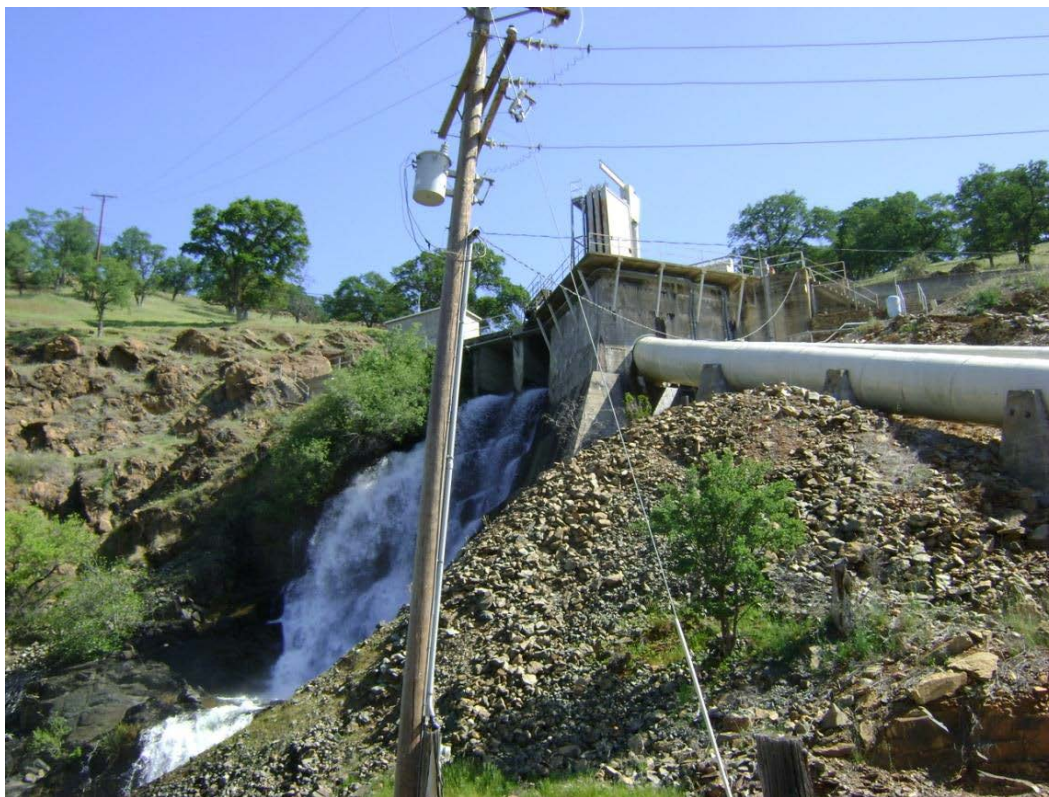
Figure 2.4-1. TID penstock intake and sluice gates. In the photo, flow is being discharged from the sluice gates to the sluice gate channel.
