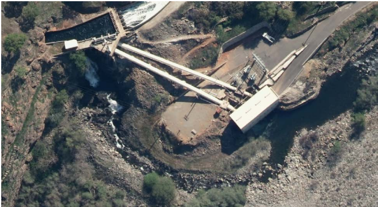
Figure B-1. Aerial photo of sluice gate channel area, forebay, penstock intakes, powerhouse and upper end of tailrace channel.
