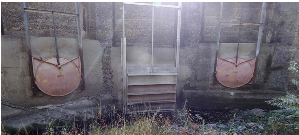
**Figure 3.0-1. Hillside gates which pass flow from the MID canal to the plunge pool below LGDD.**
