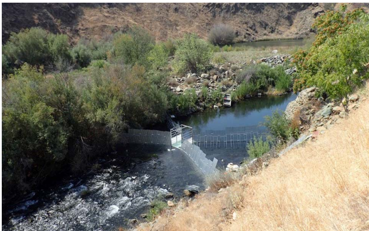
Figure 4.2-2. Overhead view of tailrace channel weir and passing chute.
