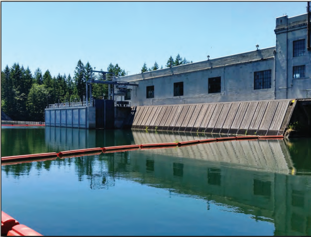
Fixed Collector, Clackamas River, OR ~ 10 ft reservoir fluctuation $12M
