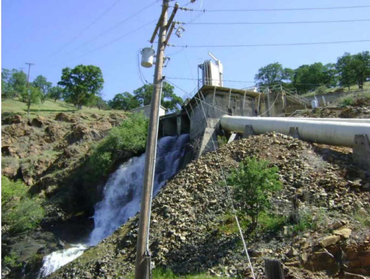
Figure 1.3-3. Sluice gate channel and penstock intake. In the photo, flow is being discharged from the sluice gates to the sluice gate channel.
